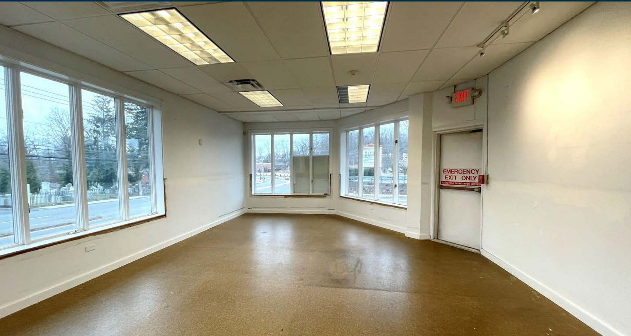
Retail Space & Emergency Exit
